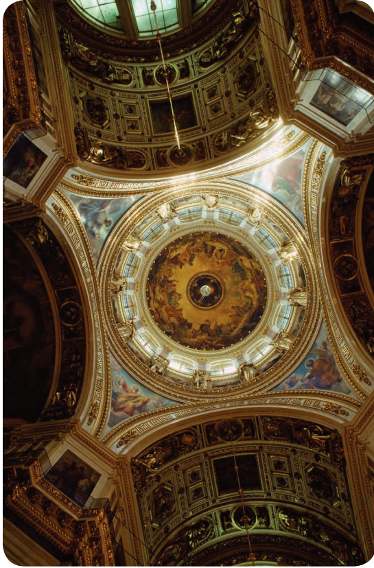
■ Figure 13 Spaces between arches set in a square to support a dome are called spandrels and are often decorative. Some features in organisms might be like spandrels, a consequence of another adaptation.
